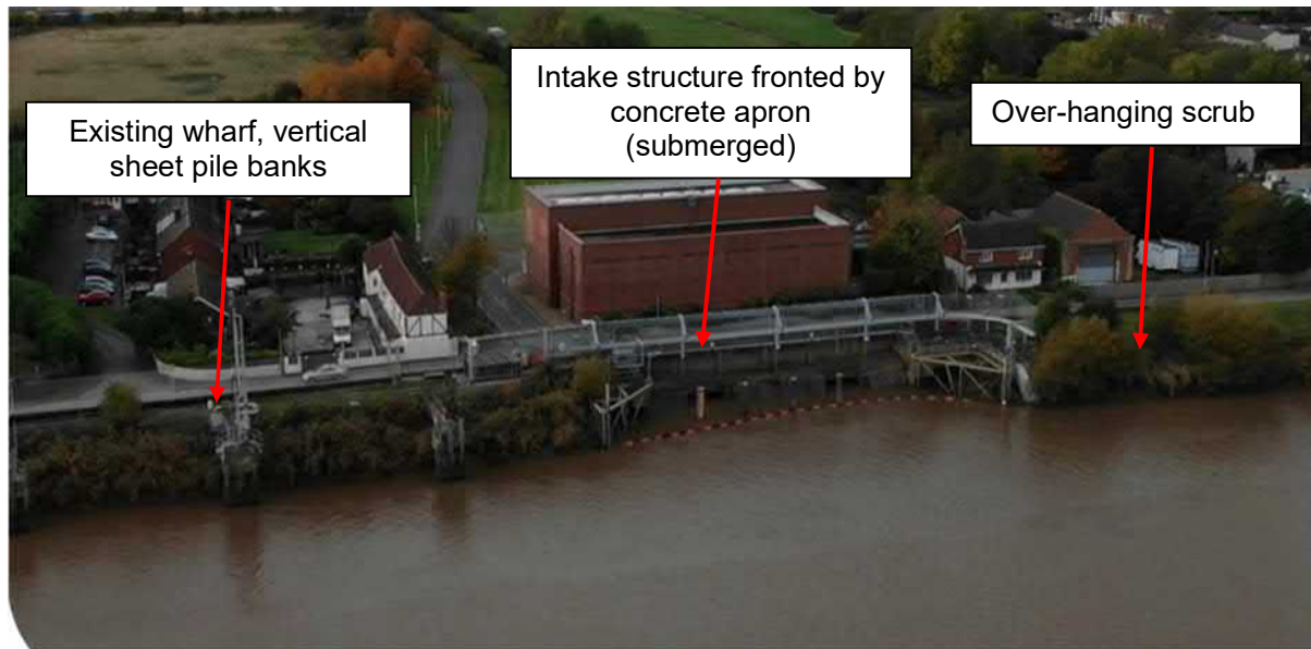
Plate 3: Location of the River Water Abstraction (Work 4B)/ existing Keadby 1 Power Station water intake structure (image taken at high tide)
